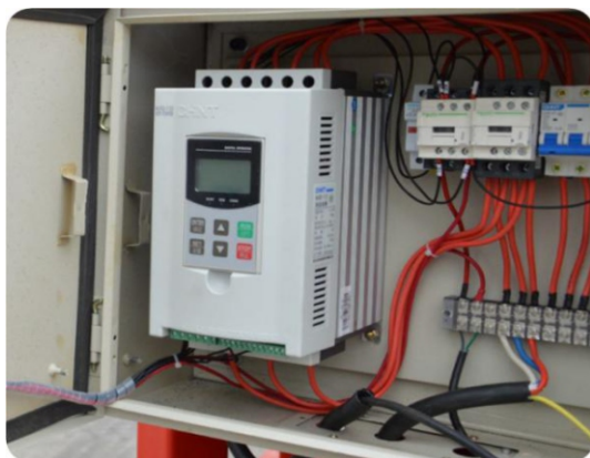
Soft start protects motor for GRM500 & GRM800
