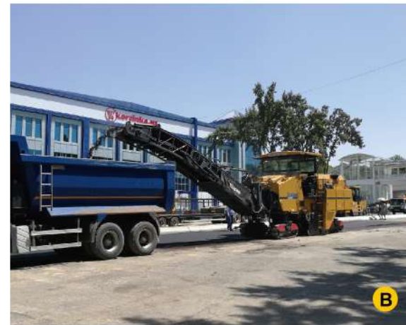
A、徐工XM503铣刨机在黑吉高速施工 B、徐工2m铣刨机在乌兹别克重要道路施工 C、延安新城徐工路拌机施工 A、XCMG XM503 was working in Heiji expressway B、XCMG 2-meter milling machine was in Uzbek city roads construction C、XM503 milling machine in Zhejiang construction
