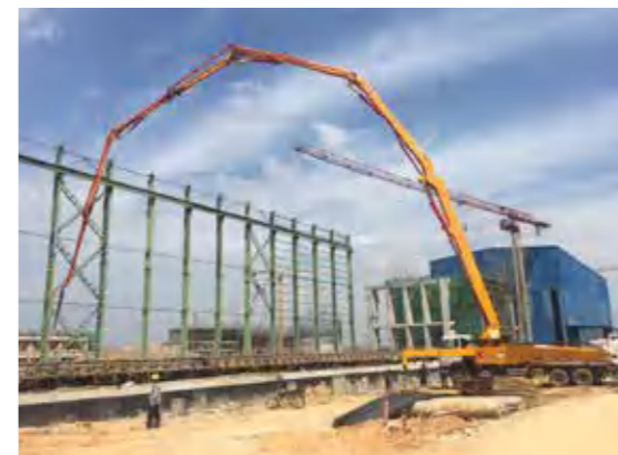
马来西亚第一台HB53K助力关丹产业园 HB53K boom pump is working in Kuantan Industrial Park of Malaysia.
