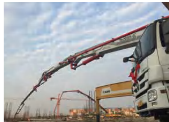
HB58米泵车展雄风 HB58K boom pump is exhibiting its manhood.
