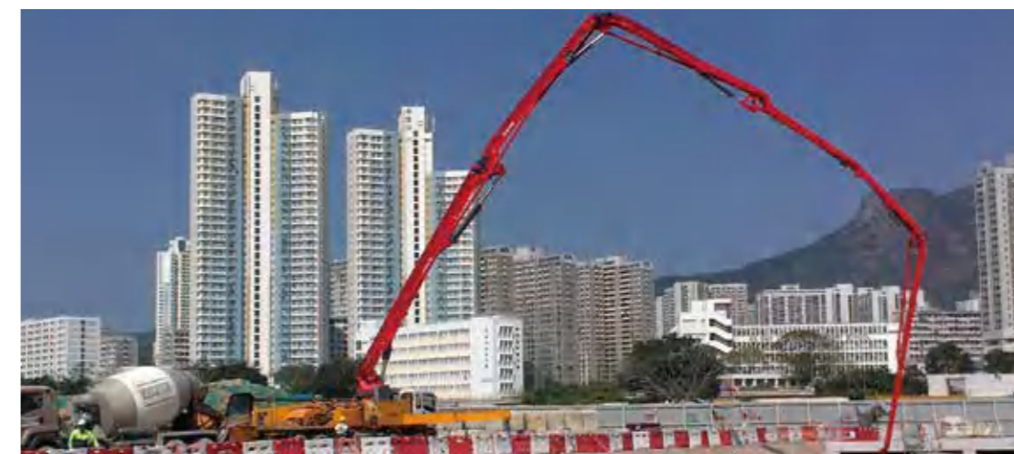
HB53K泵车香港地铁站小试牛刀 First show of HB53K boom pump at subway station of Hongkong
