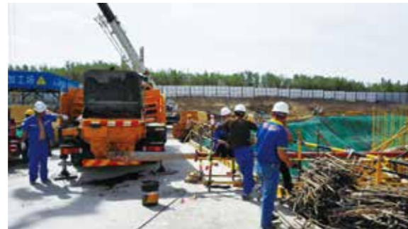
HBC10020V车载泵 新疆乌鲁木齐 HBC10020V truck-mounted concrete line pump in Urumchi Sinkiang
