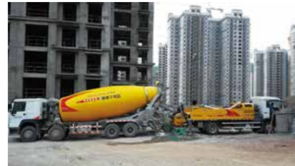
HBC10020V车载泵 新疆乌鲁木齐 HBC10020V truck-mounted concrete line pump in Urumchi Sinkiang
