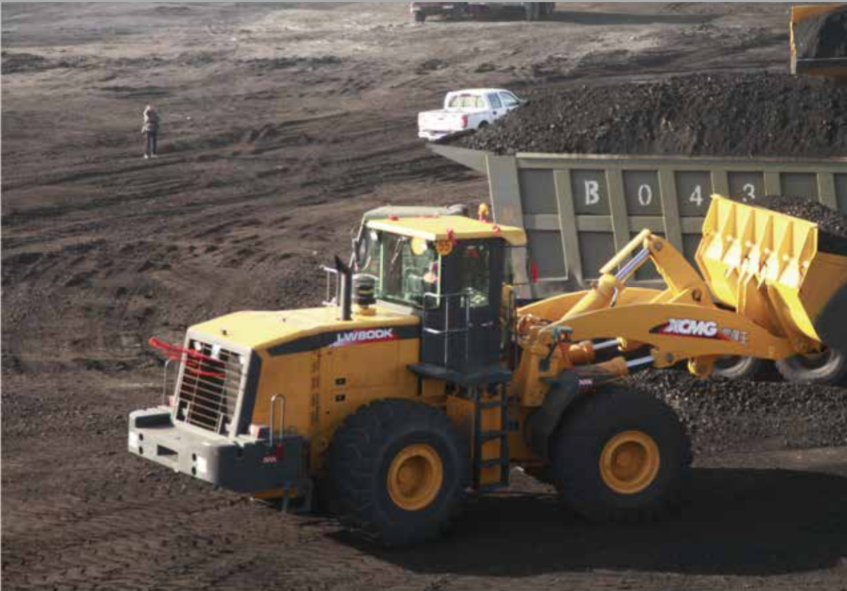
Construction scene of XCMG LW800K loaders
